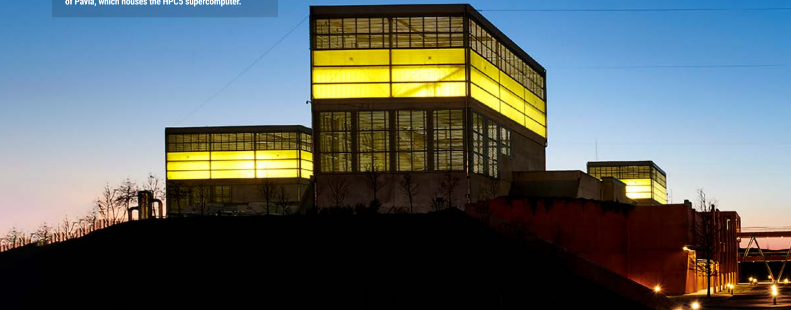
Green Data Center in Ferrera Erbognone, in the province of Pavia, which houses the HPC5 supercomputer.
